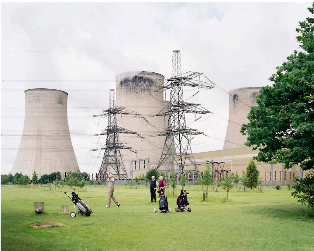
Ratcliffe-on-Soar Power Station, Nottinghamshire, 16th June 2008 [fig. 4]
