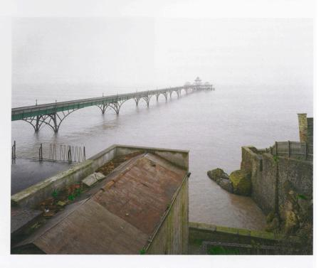
reinforced with cast iron, then wrought iron, and finally concrete. In 1940 it was more or less demolished by British soldiers in anticipation of a German invasion, and from 1946 to date, it has been continuously restored. Less typically, it was the target of an IRA bombing campaign in 1993.
