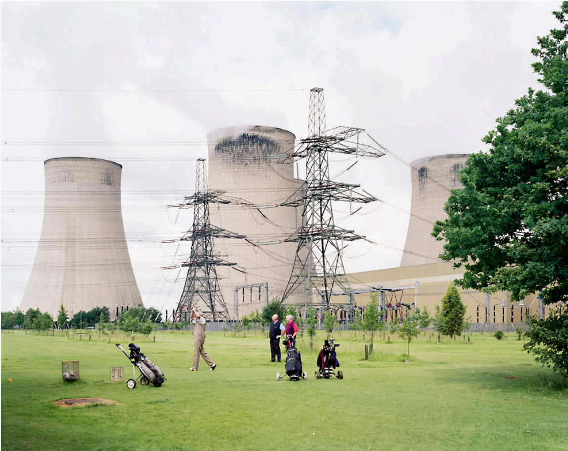
Ratcliffe-on-Soar Power Station, Nottinghamshire, 16th June 2008
